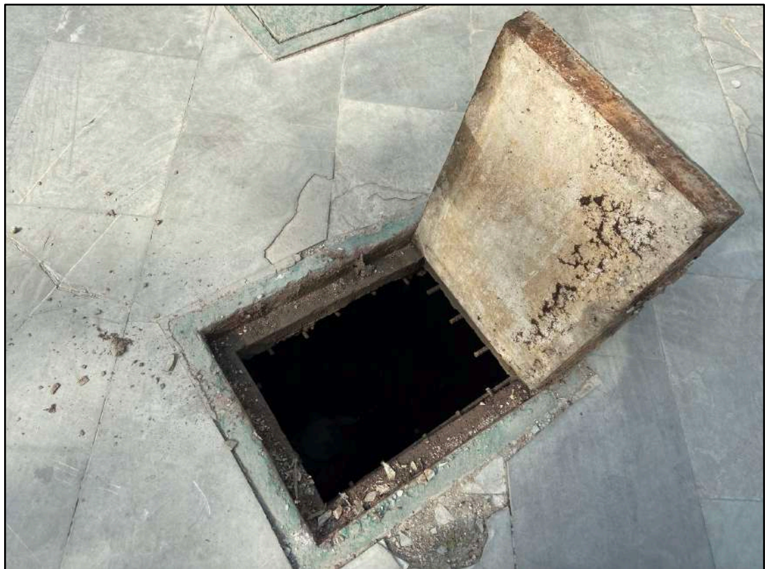
Rainwater harvesting tanks for replenishing ground water
